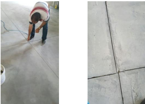
CLEAN THE SURFACE AND THE JOINT
