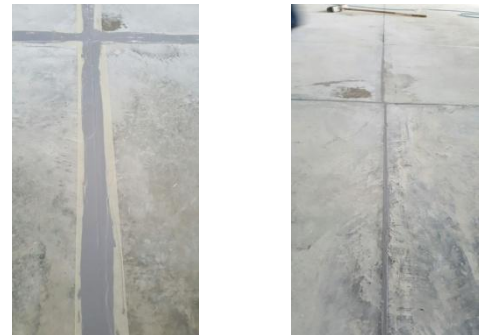
REMOVE MASKING TAPE AND THE JOINT IS SEALED
